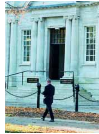
The Registry Building at University of Wales headquarters in Cardiff
