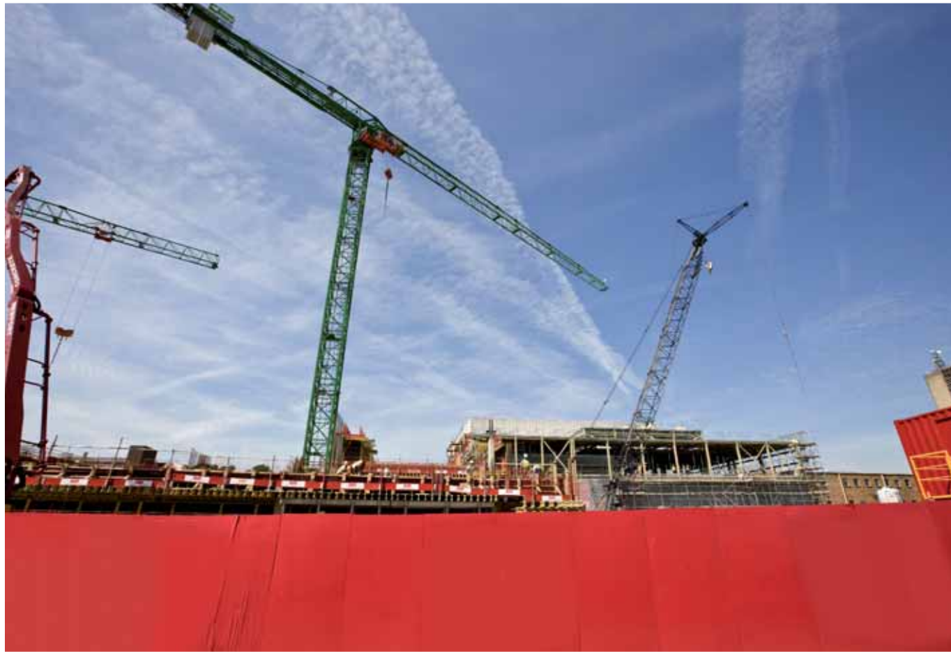
City Centre Regeneration Construction
